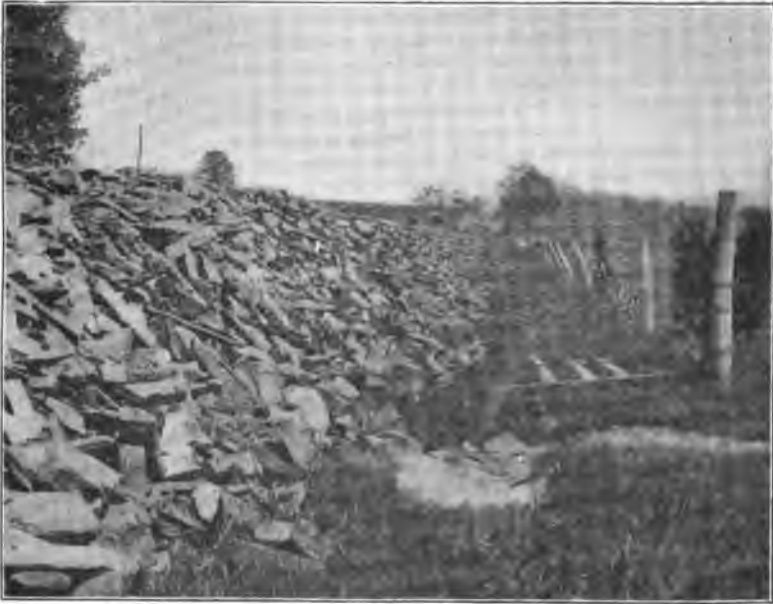
Marshall's Corner and Woodsville road, Mercer Co., showing rock fill of 12 feet.
